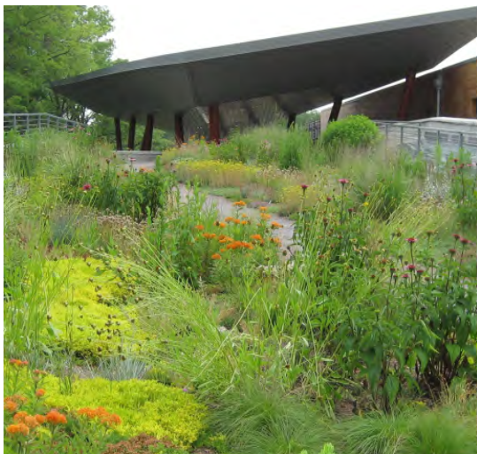
Figure 8: Intensive green roof
