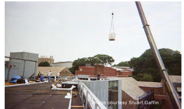
A crane delivering "super-sacks" of growing medium to the rooftop
