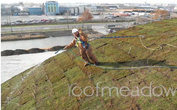
Irrigating a sloped green roof during the establishment period
