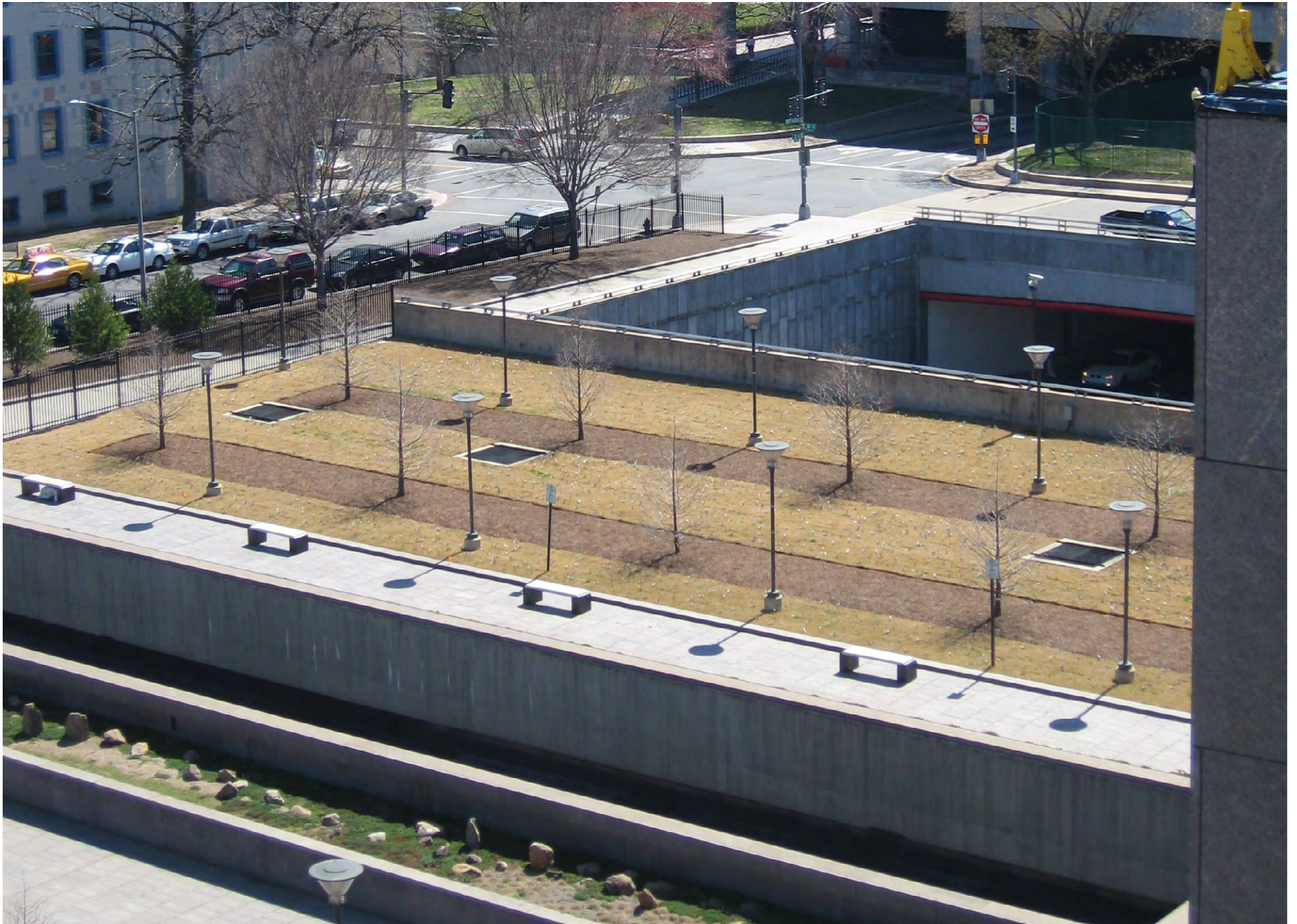
GSA National Capital Region - United States Tax Court, Washington DC A 19,600 square foot green roof installed in the plaza.
