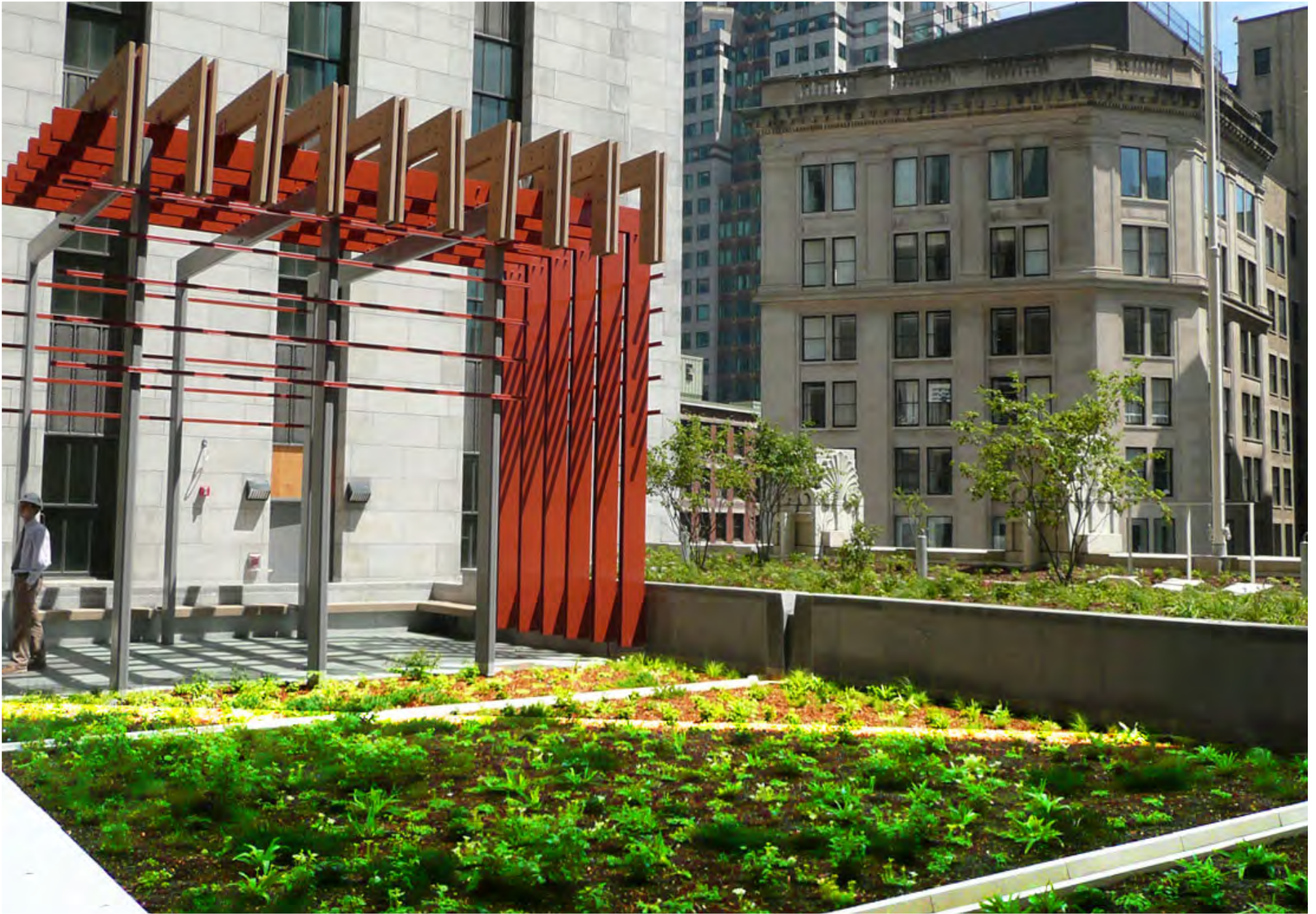
GSA Region 1 - John W. McCormack US Post Office and Courthouse, Boston, Massachusetts A 9,654 square foot extensive green roof replacing an existing, weathered roof on an this historic building (1933). The green roof is accessible by occupants and used as a filter for stormwater runoff from the surrounding, impervious rooftops.
