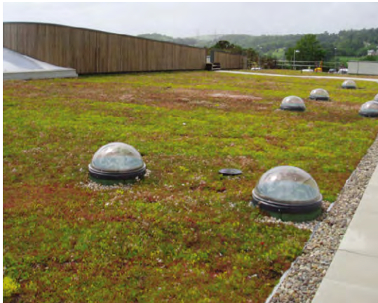
Figure 7: Extensive green roof
