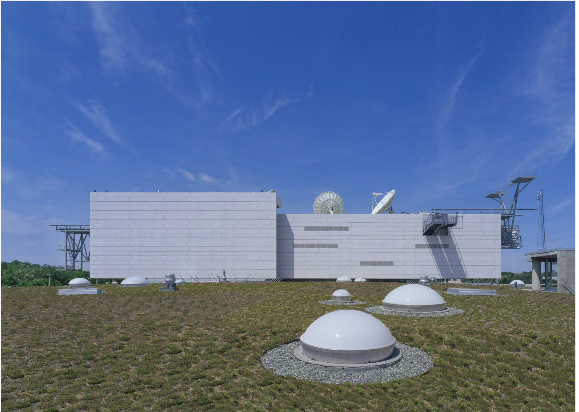
GSA National Capital Region - NOAA Satellite Operations Facility (NSOF), Suitland, Maryland A 146,000 square foot extensive green roof installed on the new LEED Gold certified operations center (2006).
