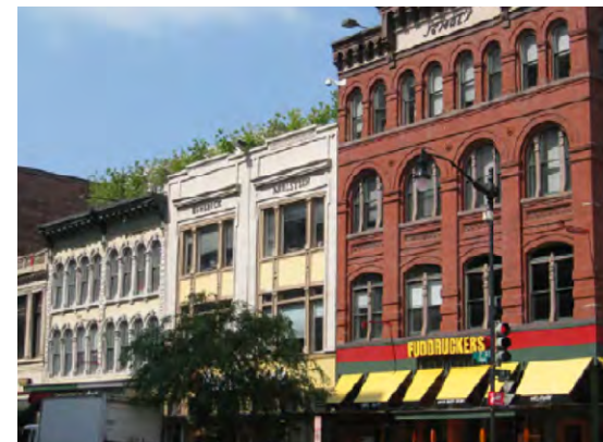
Figure 25: Incompatible green roof on a rehabilitated office/retail building
