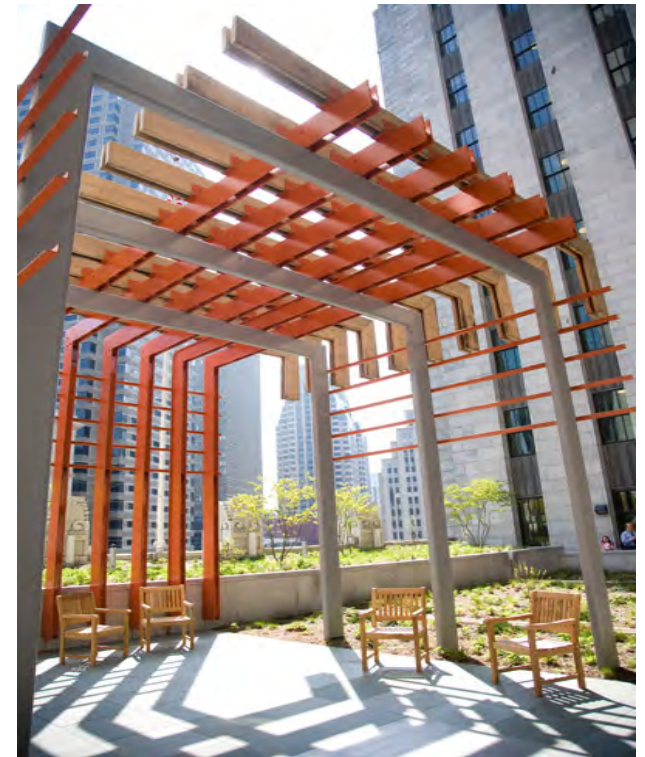
Accessible roof at the John W. McCormack Post Office and Courthouse, Boston, Massachusetts
