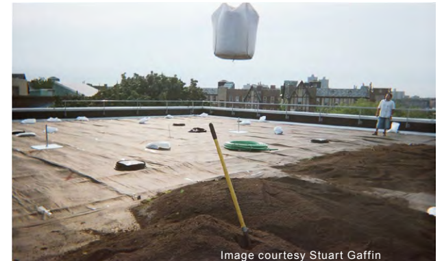
A "super-sack" of growing medium hoisted above the roof.
