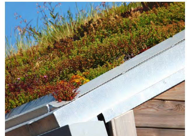
Figure 15: Sloped green roof with sedums and other plants
