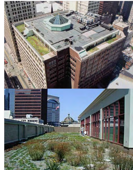
Figure 24: Compatible green roof on a rehabilitated office/retail building
