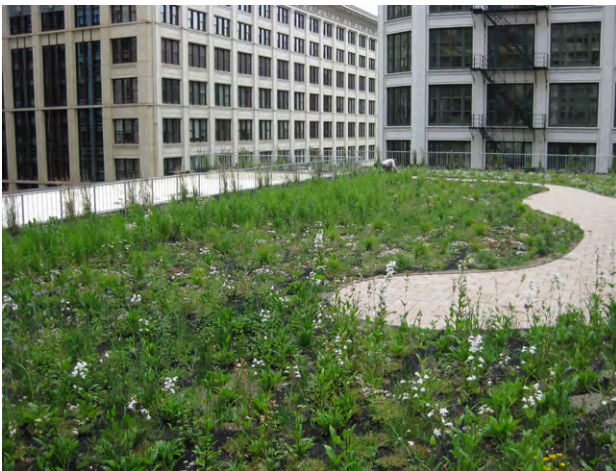
Accessible green roof at the 10 West Jackson Street Building, Chicago, Illinois
